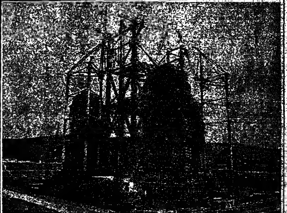
The "MAUREEN" steel gravity platform for Phillips Petroleum Co., under construction, at AMC yard
